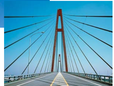
Bridge Guy Lines
